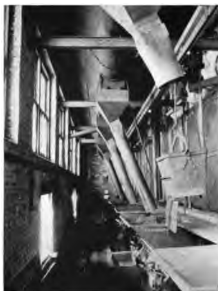
Fig. 2. Overhead Coal-Bin in which Man was Suffocated.
